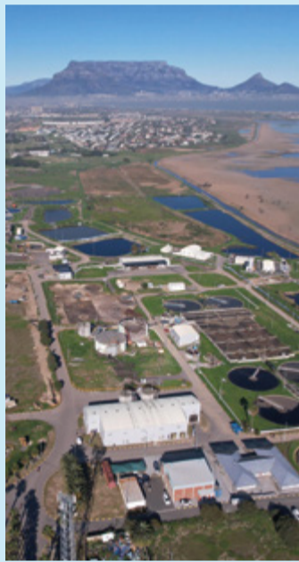
Need a bigger Pot: The R5,2 billion upgrade of Potsdam wastewater works is the second-largest infrastructure project in the Western Cape. It will double the plant's treatment capacity to 100 million litres per day and is a key step in shutting off pollution sources to Milnerton lagoon.
