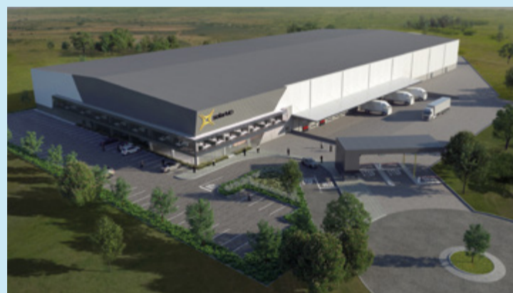
Batteries for Africa: An artist's impression of Solar MD's new Richmond Park site, which will be the continent's first dedicated plant for the manufacture of gigawatt lithium-ion battery storage. This further establishes Cape Town as a green energy hub.
