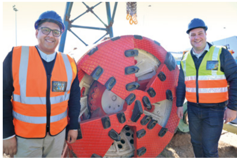
Buying in bulk: Pictured are, from left, Cllr Zahid Badroodien (Mayco member for Water and Sanitation) and Mayor Geordin Hill-Lewis on the site of the R474 million Milnerton bulk sewer upgrade project, which broke ground on 16 August.
